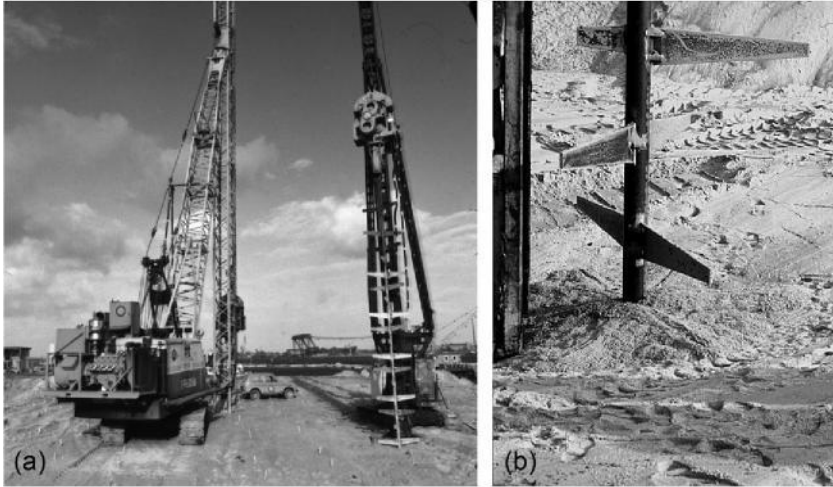
Figure 4.7 Vibro-wing equipment and compaction probe: (a) vibro-wing machine; (b) vibro-wing rod.
